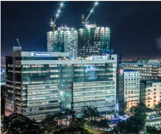
Teleperformance Bldg 18,093 sqm GLA | Cebu IT Park
