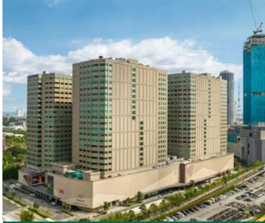
Vertis North BPO Towers and Mall 164,628 sqm, EDSA, Quezon City
