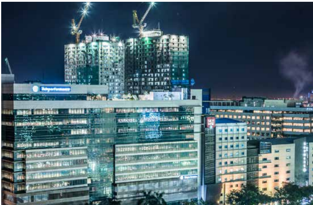
Completed in 2013, the 12-storey Teleperformance Cebu is located in the 27-hectare Cebu I.T. Park.
